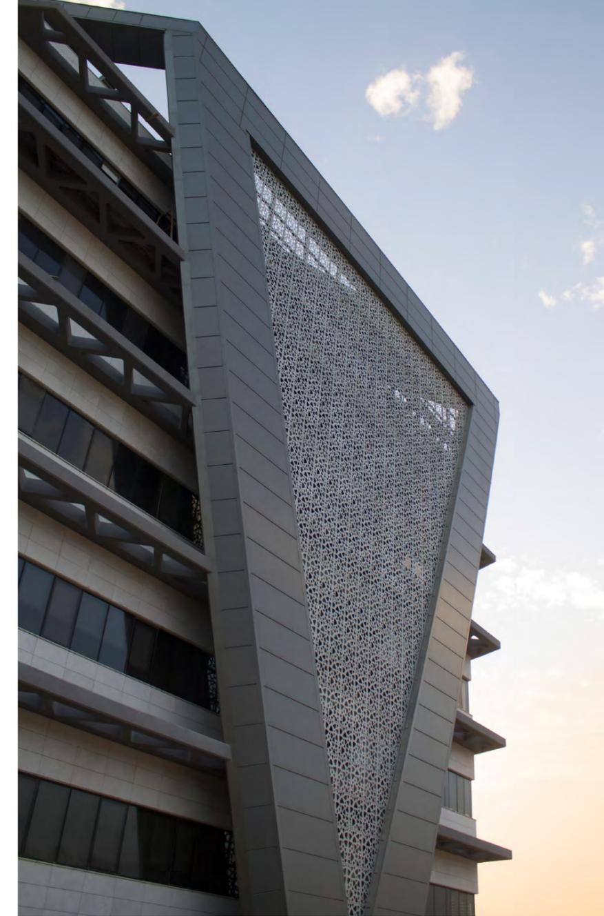
Ramallah is known for its mediterranean climate with cold winters and long, warm and dry summers with average daily temperature above 25°C, which is why the Qbiss One facade system was also the best choice thanks to its insulation properties. With mineral wool insulation it can achieve a high thermal insulation level with U values up to 0.16 W/m<sup>2</sup>K and contributes to thermally pleasant and stable interior climate.
