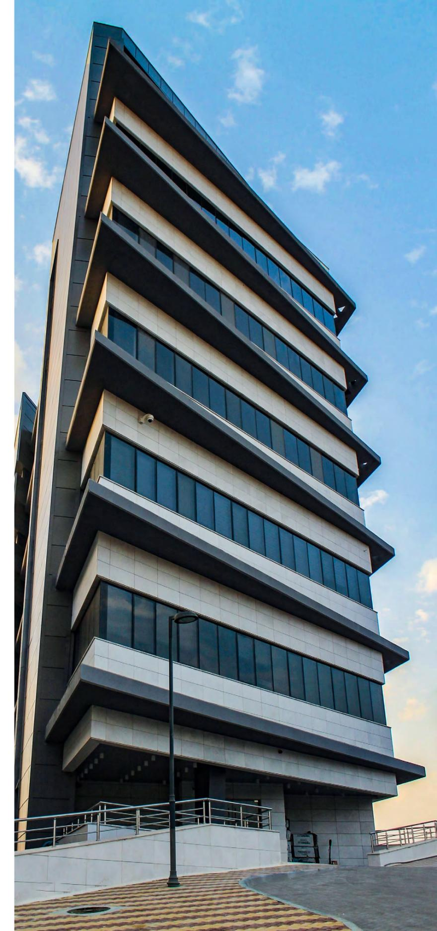
The dynamic of the horizontally assembled façade is created by alternating local stone cladding and slightly overhanging assembled Qbiss One elements.
