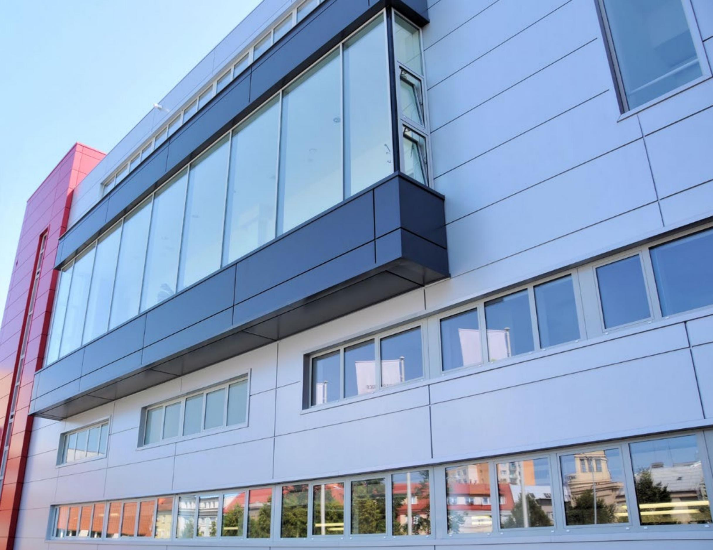
▀▀ In spite of the fact that these type of projects usually use built-up systems, we decided on Qbiss One because of the very aesthetical outer look of the facade, especially the details in crossing of the joints. There were three different colours chosen for this project because it is a very large building and we didn't want to have it in just one colour shade.
