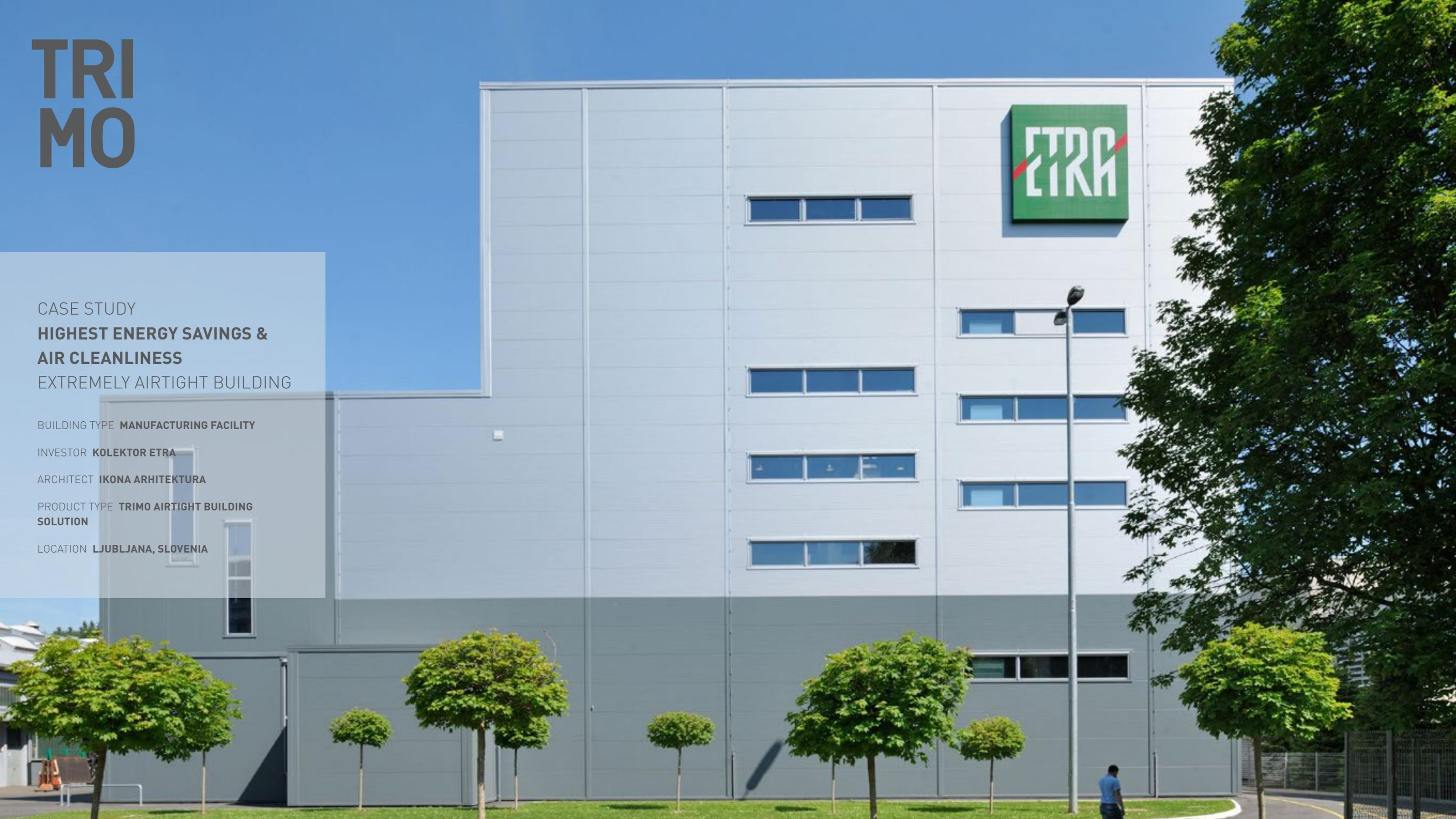
A high level of **air cleanliness**, low and controlled humidity were basic client requirements for a new production facility for the large electrical power transformers. **Trimo's highly airtight building system** was an ideal solution for the clients needs. The building is extremely airtight and economic in use as it facilitates **low energy consumption**, which brings substantial energy savings.
