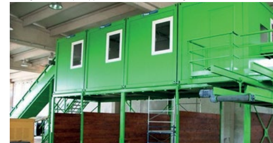
Waste Treatment Center, Krk, Croatia
