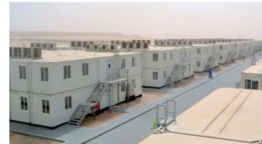
Remote Site Camp, Al Wasita, UAE
