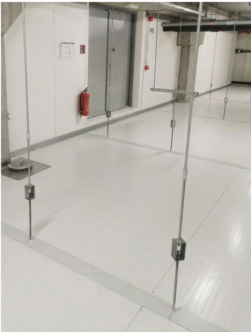
Fig. C4.1: Trimoterm ceiling from above.
